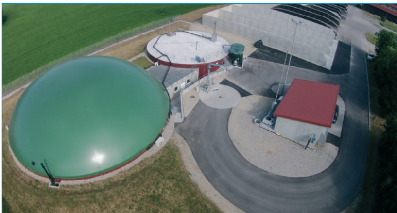
Fig. 5: Demand-oriented electricity generation is tested on the biogas plant of the Bavarian State Research Center for Agriculture in Grub (near Munich) ■
