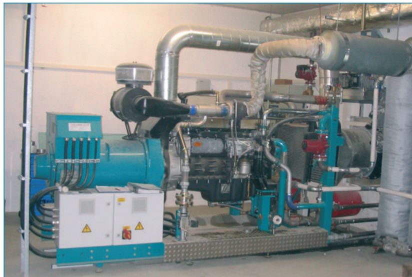
Fig. 2: View of a biogas driven co-generation unit with reciprocating engine (center) and generator (left side; Photo: LfL) ■
